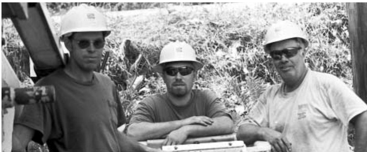
From left, Gene Manning, Shane Blake and Bob Fair take a break while setting poles for a new line extension.
