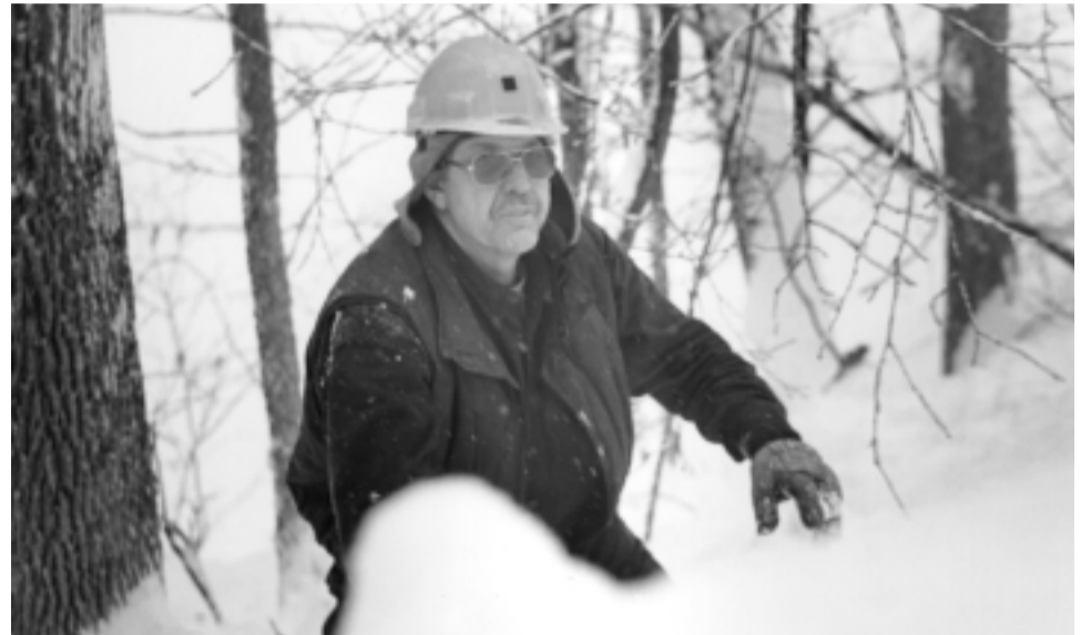
Lineman Dennis Bador struggles in waist-deep snow up an embankment in Moretown.
