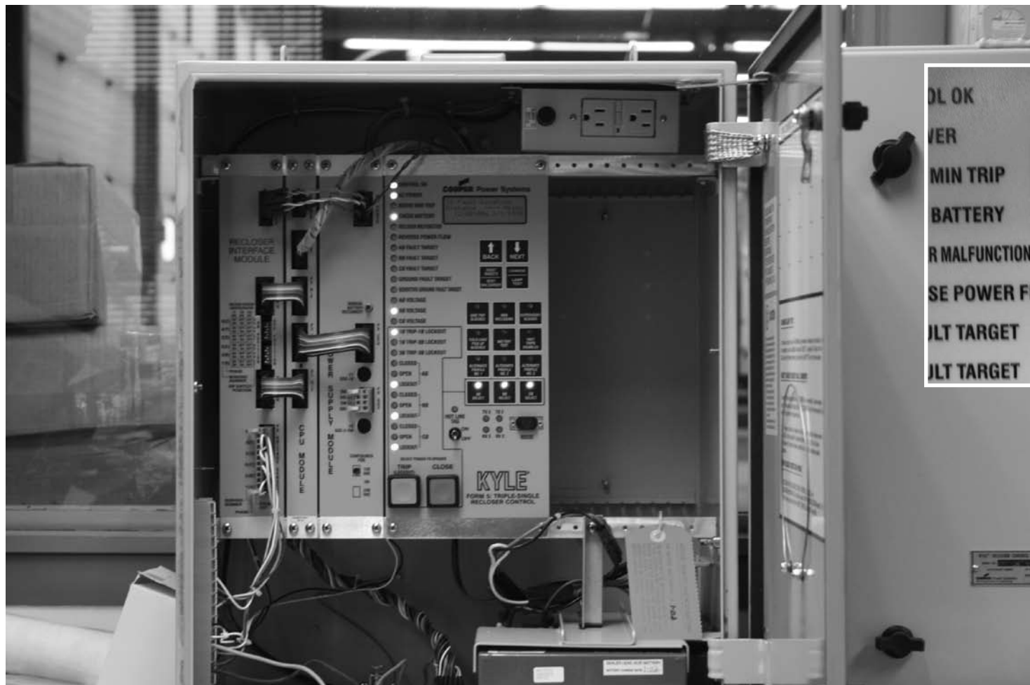
At left, the insides of a Nova vacuum recloser like those shown at the substation on page one. It conveys a lot of information, but one of the most interesting things is the screen (on the right side of the display, and magnified in the photo above), which can tell the operations workers how far away from the substation a fault has occurred. Remarkably accurate, this information cuts down on searching for the source of an outage.
