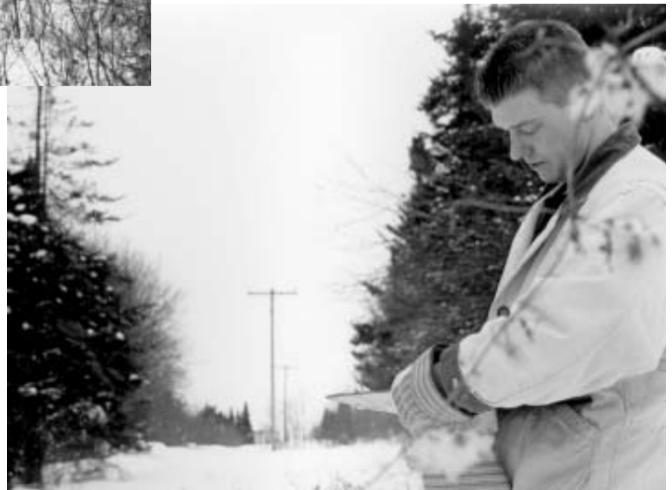
(Top left) It's time to modernize some of WEC's earliest line, like this stretch in Williamstown where a 1940-vintage pole inclines to the right. (Above) Kevin Stevens takes measurements at a site destined for an upgrade this summer.
