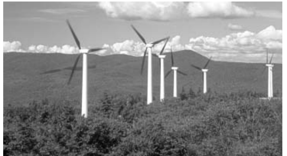
Green Mountain Power Corp.'s wind farm at Searsburg. These towers, which stand 130 feet tall, are much smaller than newer models of utility-scale wind turbines.
