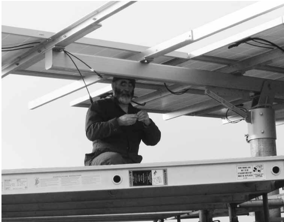
Ed Hutchinson installing and wiring one of the family's two 2,500-W, pole-mounted PV arrays (above and below). It's the two pole-mounted systems that are tied into the grid and, converted from DC to AC power, contribute to the Co-op's electricity network. Photos courtesy of Ed Hutchinson.
