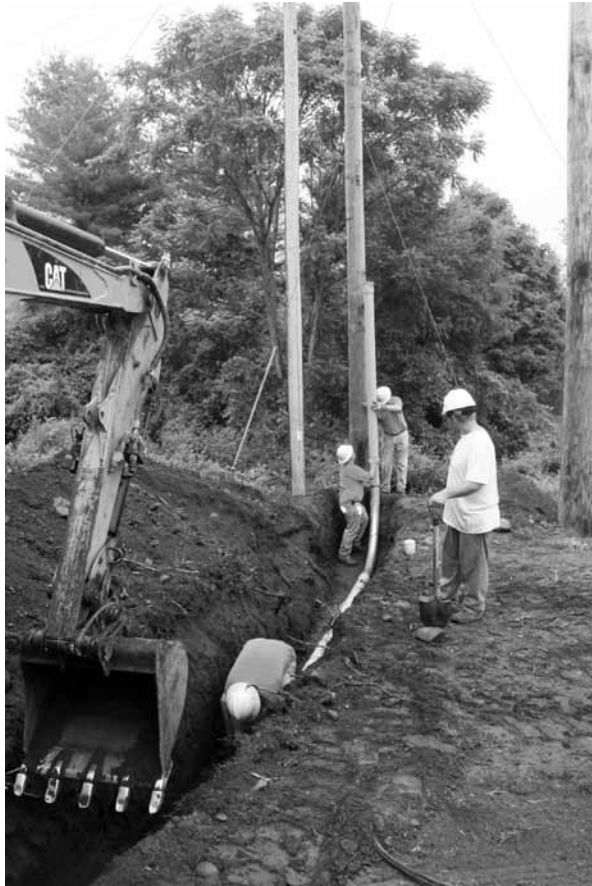
The barren site where Washington Electric Co-op’s East Montpelier substation once sat (below) is being prepared to host a new state-of-the-art substation, to improve service and power quality for WEC members in numerous ways. At right, WEC linemen prepared a trench for conduit into the new facility.
