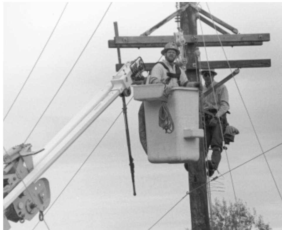
Project Foreman Bob Fair, above on left, and Apprentice Raymond Hall wrestle a piece of equipment to the ground, while (right), Linemen Richard Hallstrom, left, and Larry Brassard make connections to a new distribution-line pole that will send power out to Duxbury-area WEC members.
