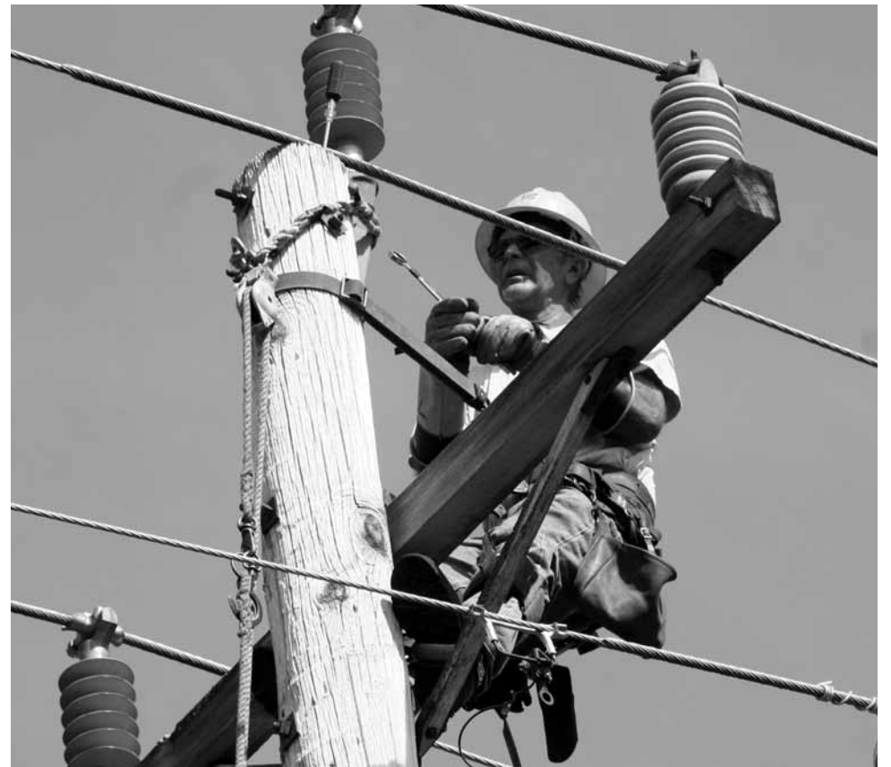
The insulators being replaced along an 8.2-mile transmission line are the spirally devices mounted on the poles and cross arms. With age, several of the insulators have cracked, which can cause an outage or even a pole fire if the energized wires contact the wood. Above left, Class A Lineman Hans Pope-Howe mounts a pole in East Montpelier to begin replacing them, while a few poles away on the same line Foreman Tim Pudvah is doing the same job.
