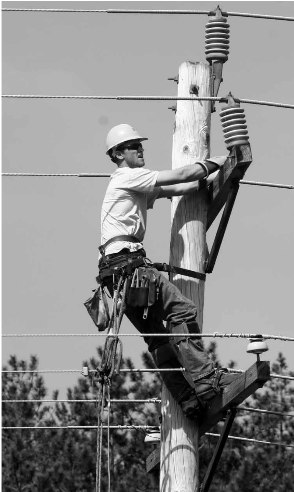
The insulators being replaced along an 8.2-mile transmission line are the spirally devices mounted on the poles and cross arms. With age, several of the insulators have cracked, which can cause an outage or even a pole fire if the energized wires contact the wood. Above left, Class A Lineman Hans Pope-Howe mounts a pole in East Montpelier to begin replacing them, while a few poles away on the same line Foreman Tim Pudvah is doing the same job.
