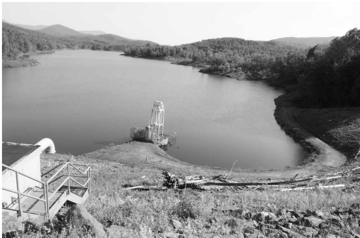
The Wrightsville Reservoir, two weeks after the flood. The line of debris in the foreground reveals how amazingly high the water line was at its pinnacle in May – far too high for operating WEC's power station.
