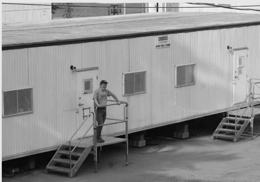
WEC's new, temporary, office building – a doublewide trailer designed with office space inside – was installed in the parking lot on Monday, June 6. For Manager Avram Patt, pictured on landing, a clean and fresh workplace was a welcome change.
