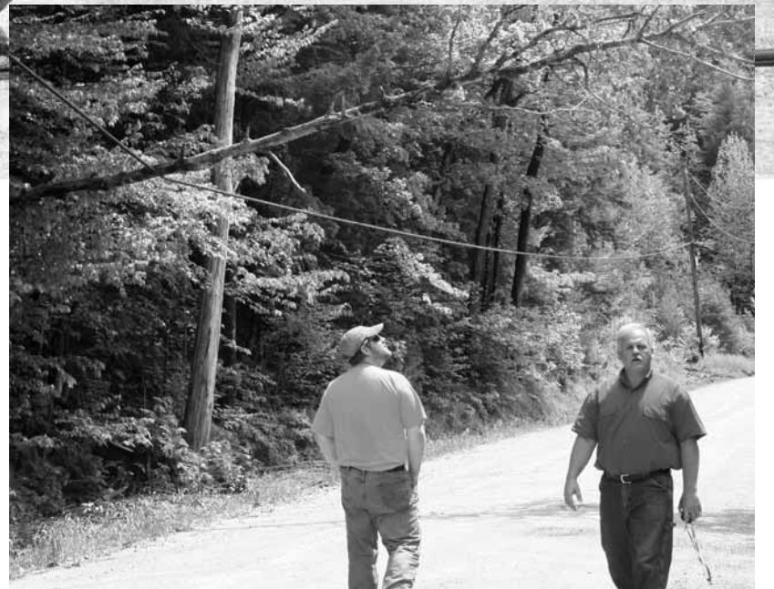
WEC Operations Director Dan Weston (left, above) and Maintenance Foreman Rich Hallstrom survey the damage to the Co-op's poles and wires on Brook Road in Plainfield. They had to walk to the site because the road was barricaded to traffic. At right, a broken tree lies across the conductors.
