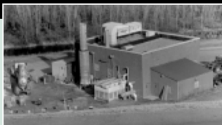
The power station tucked below the landfill is where methane makes electricity.
