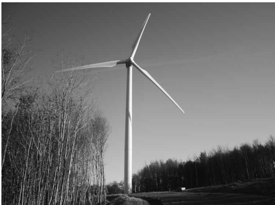
The towers are 275 feet tall, but the blades, at full extension, reach 420 feet into the air. Yet the turbines can look deceptively small from some angles.
