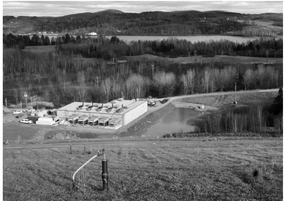
The view from a summit at the NEWS-VT landfill. That's a well cap in the foreground, which enables landfill employees to monitor the biological processes underground, and the South Bay of Lake Memphramagog in the distance. In the middle is WEC's generating station, fed by landfill methane. It provides most of your electric power.
